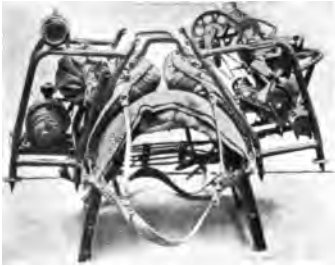
a. Generating plant (packed).
